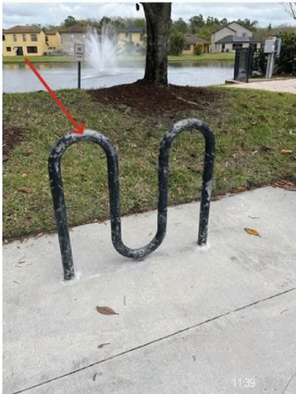
Issue 22 - Savannah Park Dr. Assigned To Inframark The bicycle parking rack needs paint.
